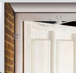
White stays hold the door in the open position preventing slam closure in windy conditions
