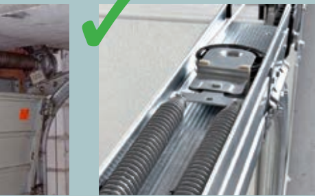
Concealed springs shown from above with the covers removed.
