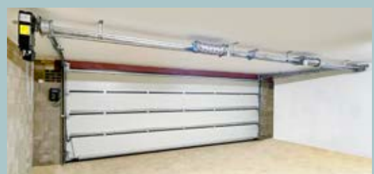
Low headroom rear torsion spring option.
